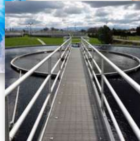
Potable Water Treatment
